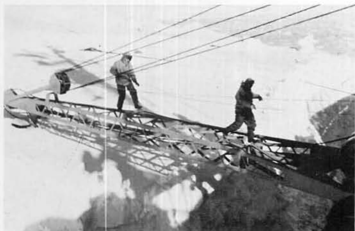
(right) for temporary gangway until permanent one can be constructed for unloading to Weddell Sea ice shelf.
