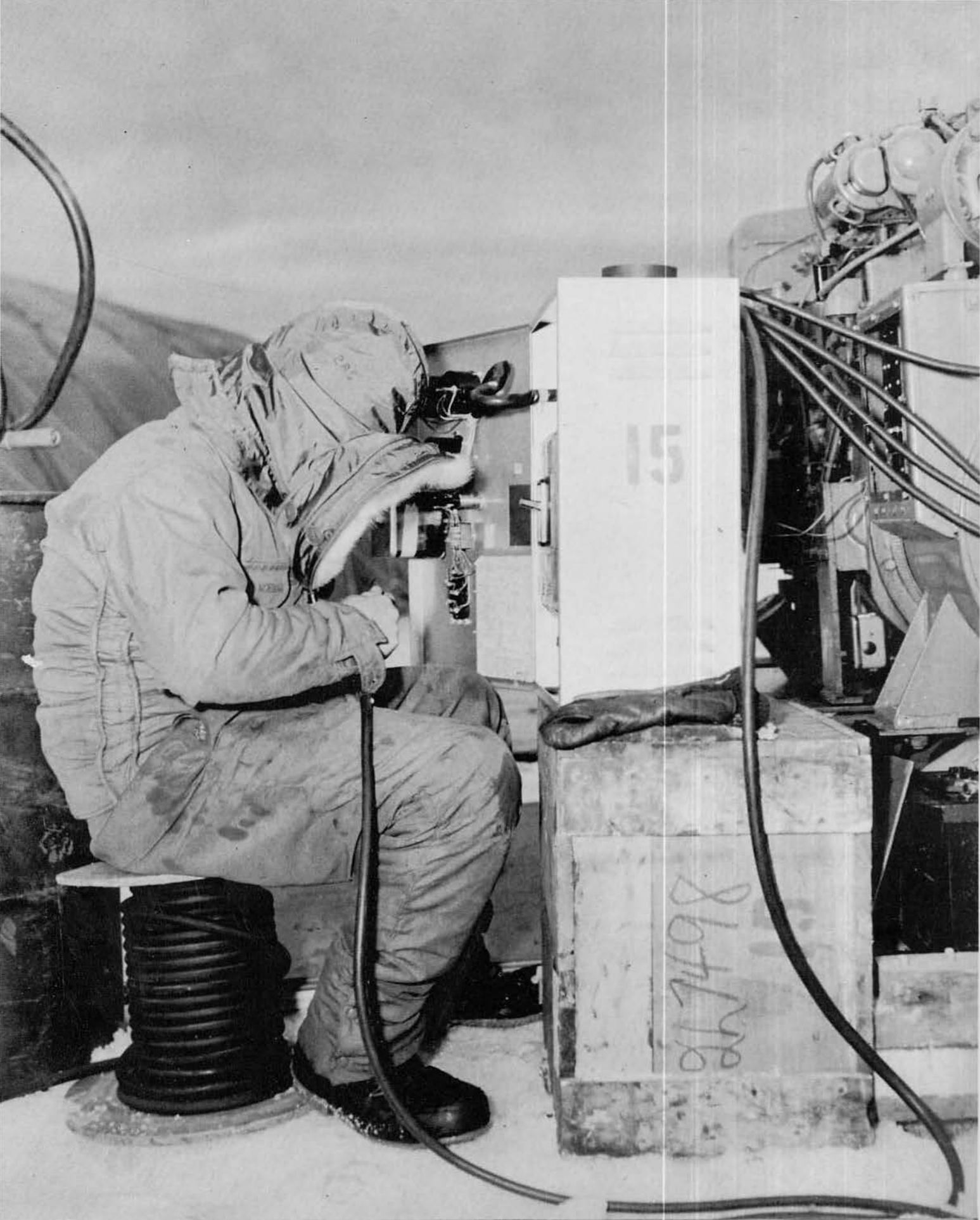
LOOKING LIKE A "SUNBONNET BABY" SEABEE ELECTRICIAN HOOKS UP GENERATOR AT WILKES STATION.
