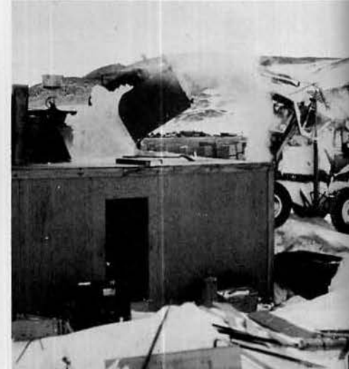
HARVESTING SNOW FOR THE MELTER HAS BEEN REDUCED TO A SCIENCE THANKS TO PARACHUTE BAGS AND TRACTORS.
