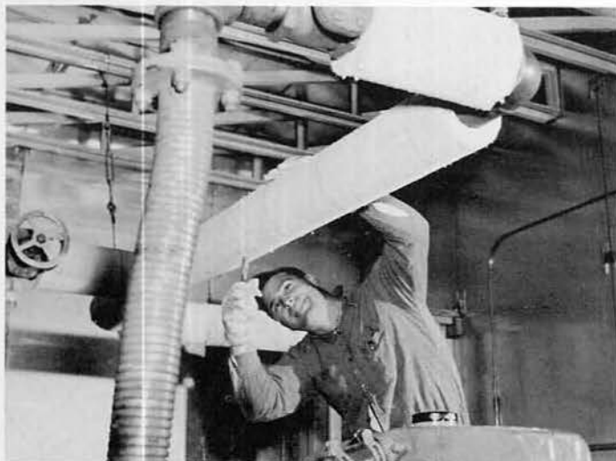
INSULATING PIPES LEADING TO BASE SNOW MELTER.
