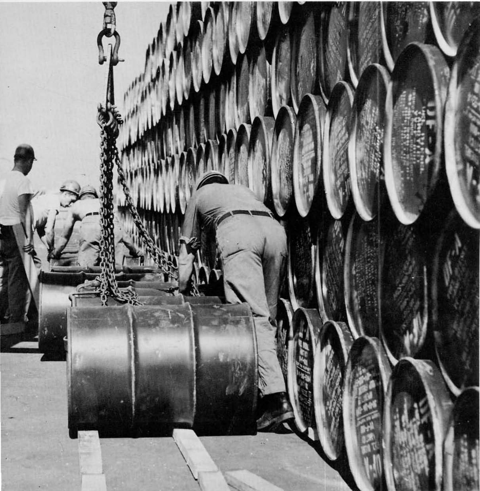
DRUMS OF FUEL ARE STACKED FOR ONLOADING AT DAVISVILLE IN PREPARATION FOR VOYAGE SOUTH.
