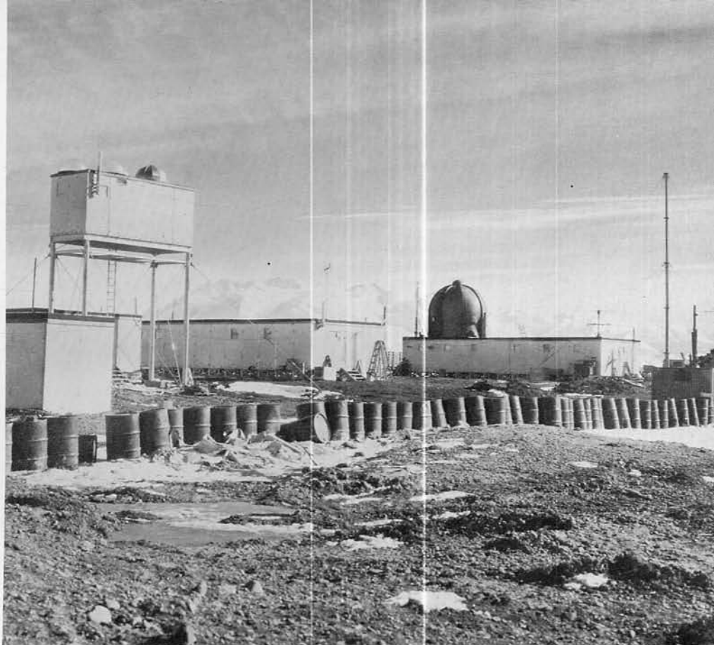
AURORA AND RAWIN TOWERS AT HALLETT WITH PENGUIN-PROOF FENCE.
