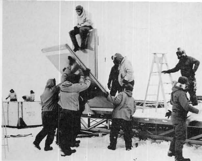
SEABEES RAISE WALL PANELS OF HUT INTO PLACE.
