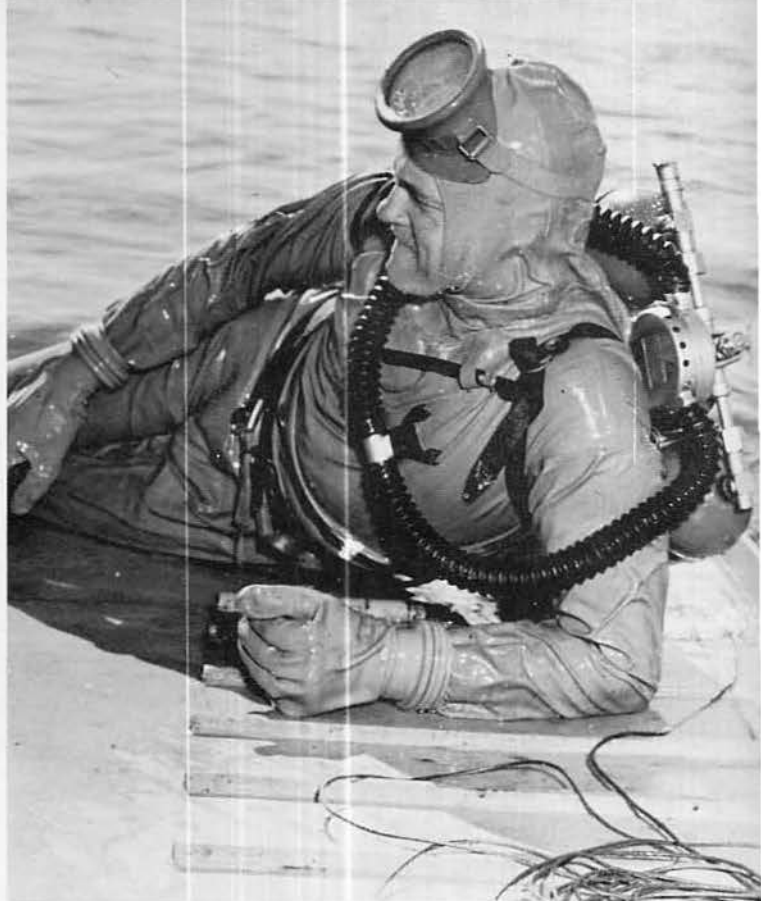
UDT MAN CHECKS NORTHWIND'S BROKEN PROP.
