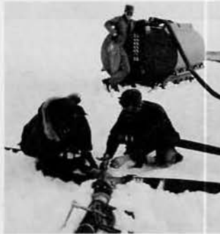
fuel lines and booster pumps are hooked up to transfer gas and fuel from both ships and the from the frozen-in YOG.
