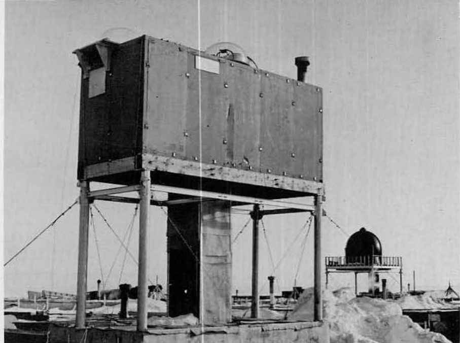
AURORA TOWER (right) at LA-V has glass domes from which weather and other conditions can be observed during winter in comparative warmth and comfort (as above).
