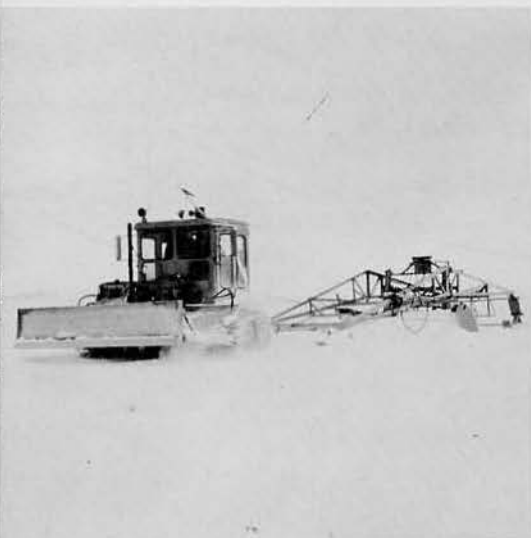
RUNWAY REPAIRS ARE MADE BY LEVELING WITH LAND PLANER, FILLING GOUGES, CHECKING STRESS POTENTIAL OF ICE.
