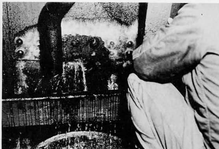
BEAT-UP WYANDOT SHOWS SCARS: CRACKED SEAM (LEFT), BROKEN PROP BLADES ARE PHOTOGRAPHED.
