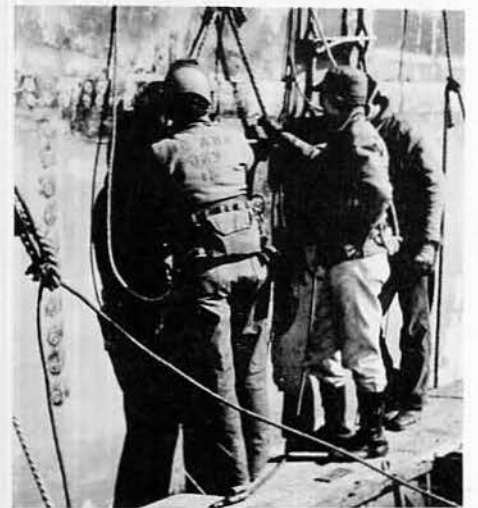
move ice from ARNEB's bow with propeller wash. Purposely created port list brings damaged hull above water for repairs (lower center) by damage control party on scaffold. ARNEB lived to fight another ice crusher off Hallett!
