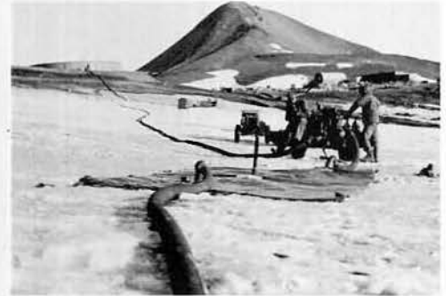
fuel lines and booster pumps are hooked up to transfer gas and fuel from both ships and the from the frozen-in YOG.
