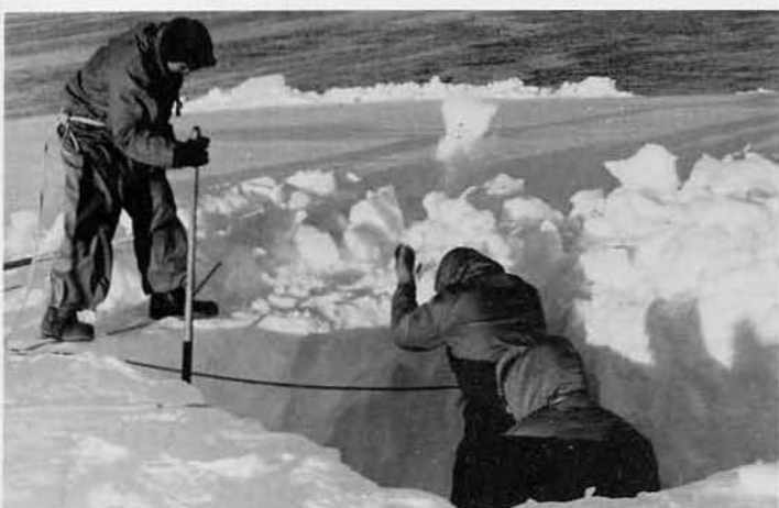
WYANDOT lies to while crewmen dig holes for deadmen (top and lower left). STATEN ISLAND lowers its crane
