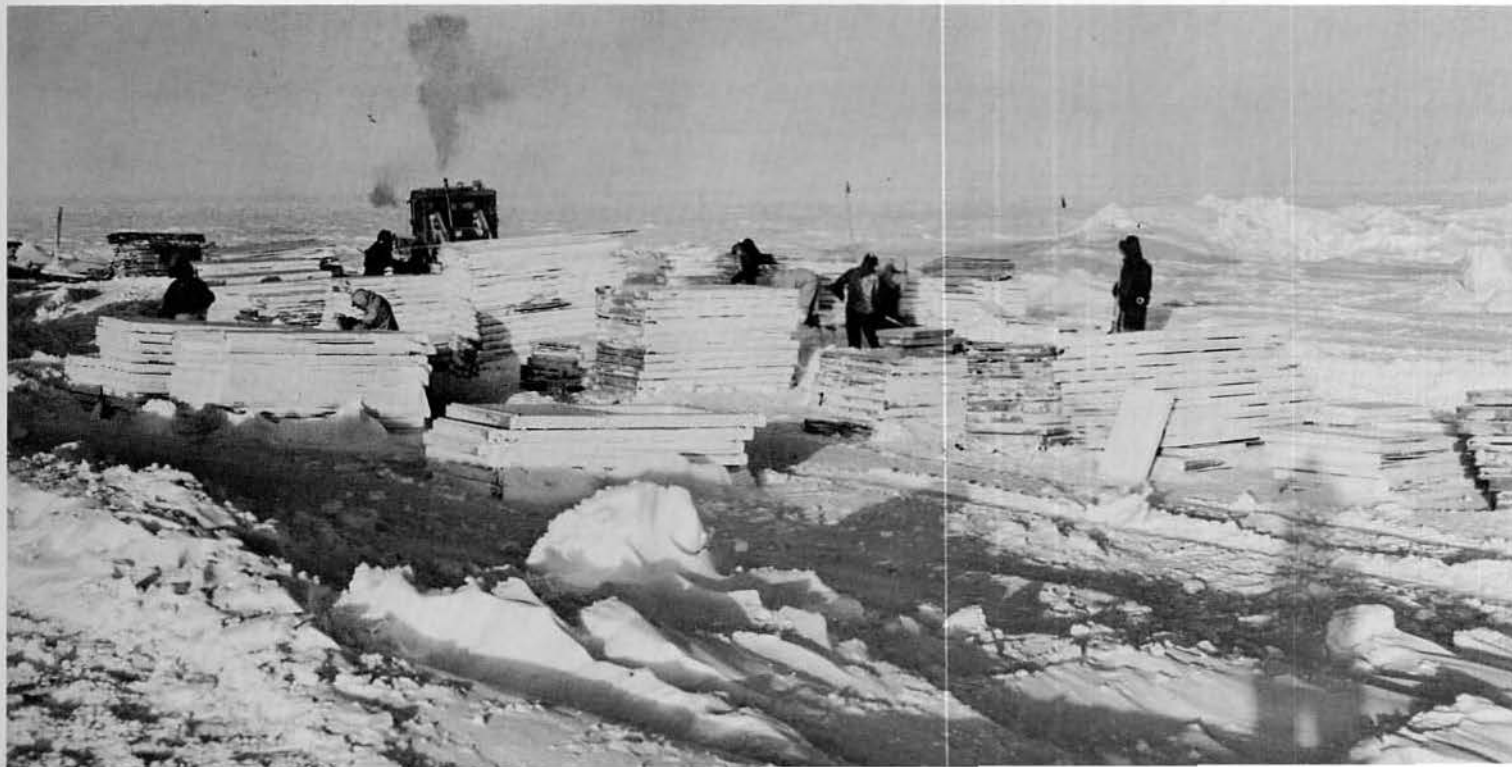
CWO VICTOR YOUNG (RIGHT CENTER) KEEPS AN EYE ON THE TRACTOR TRAIN AND ON THE CREVASSE-RIDDEN TRAIL . MCB (SPECIAL) MEN WORK ON BUILDING PANELS THAT WILL BE RAISED TO FORM PERMANENT BYRD STATION .
